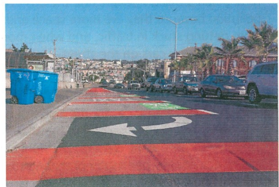
Red transit lanes are often dashed approaching intersections to make it easier to know where to enter the lane before making a turn.
