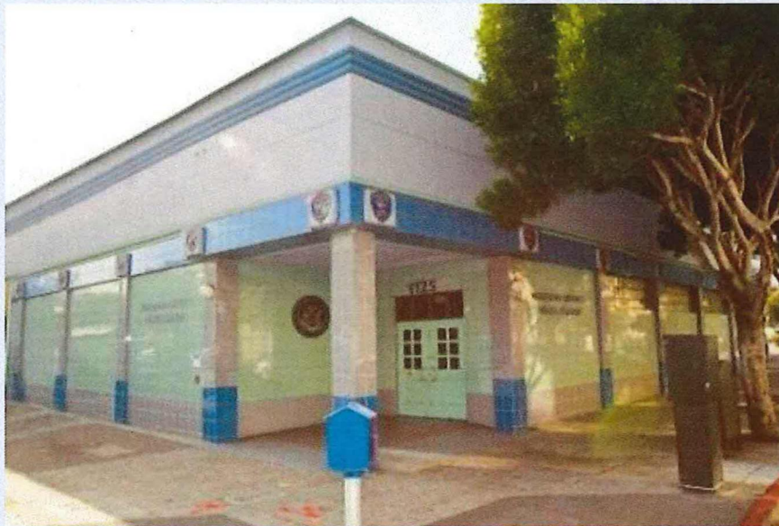
Northern Police Station Turk / Fillmore
